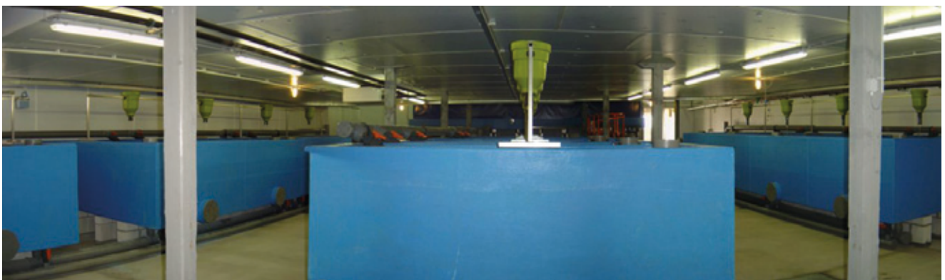
Aquakultur-Kreislaufanlage Aquaculture closed-circuit facility
